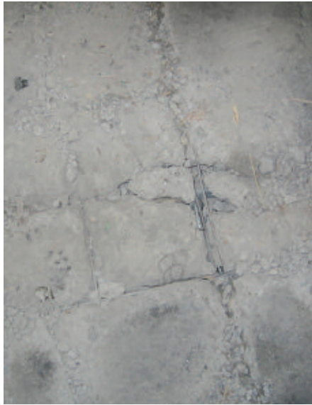
Concrete mezzanine flooring with significant damage prior to ResinDek
