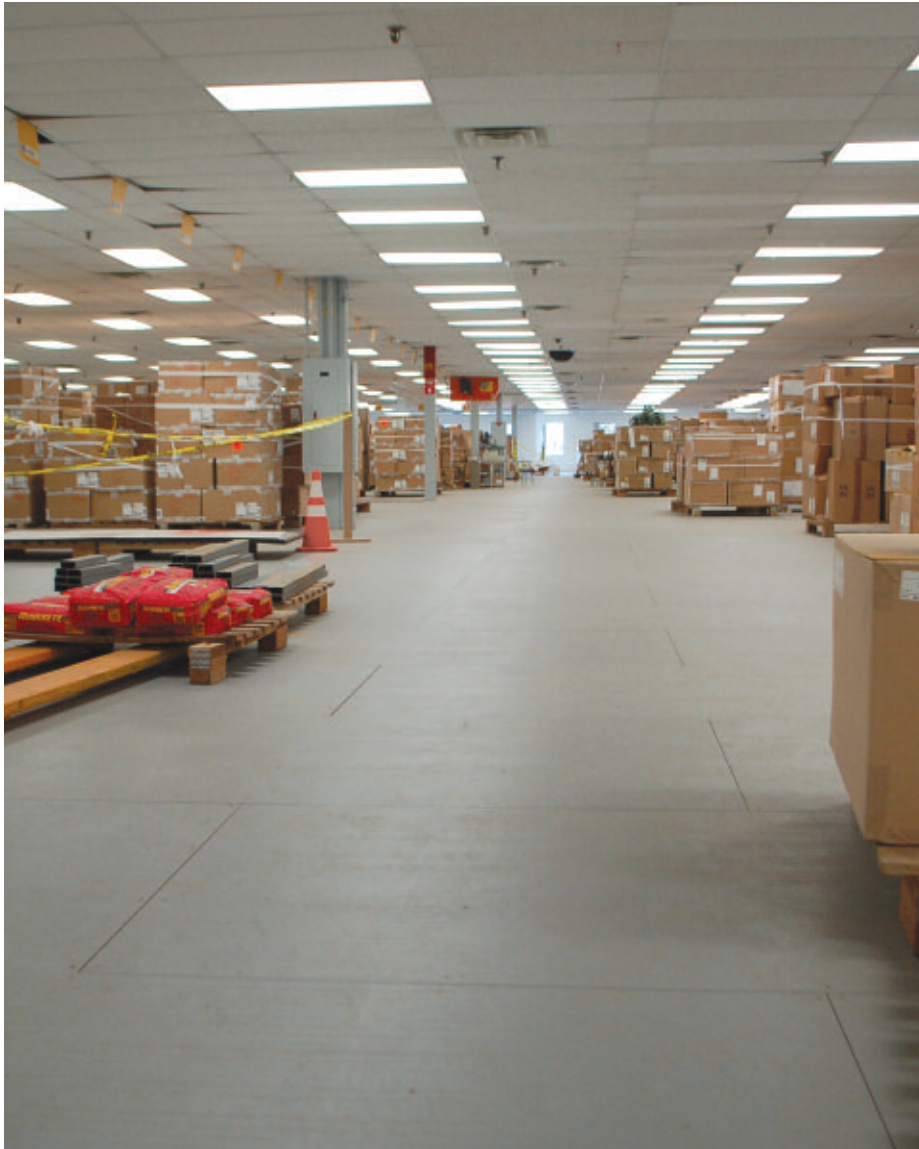
New ResinDek® panels installed
