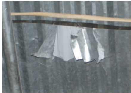
Attempted repairs beneath the mezzanine to block debris from falling through
